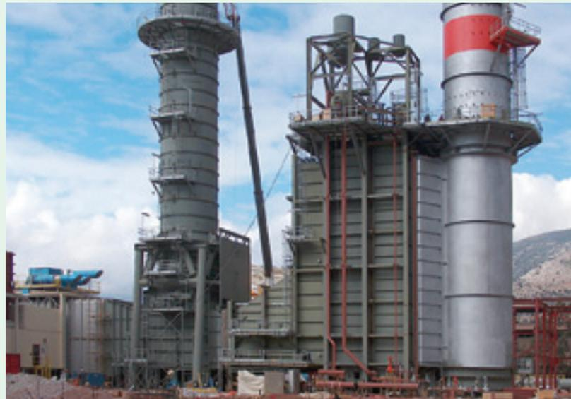
Baltec gas-turbine exhaust and heat recovery system
